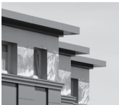
Long-term renewal and maintenance with cost-effective modernisation using ALUCOBOND®: Höxterstraße in Hagen, Germany
