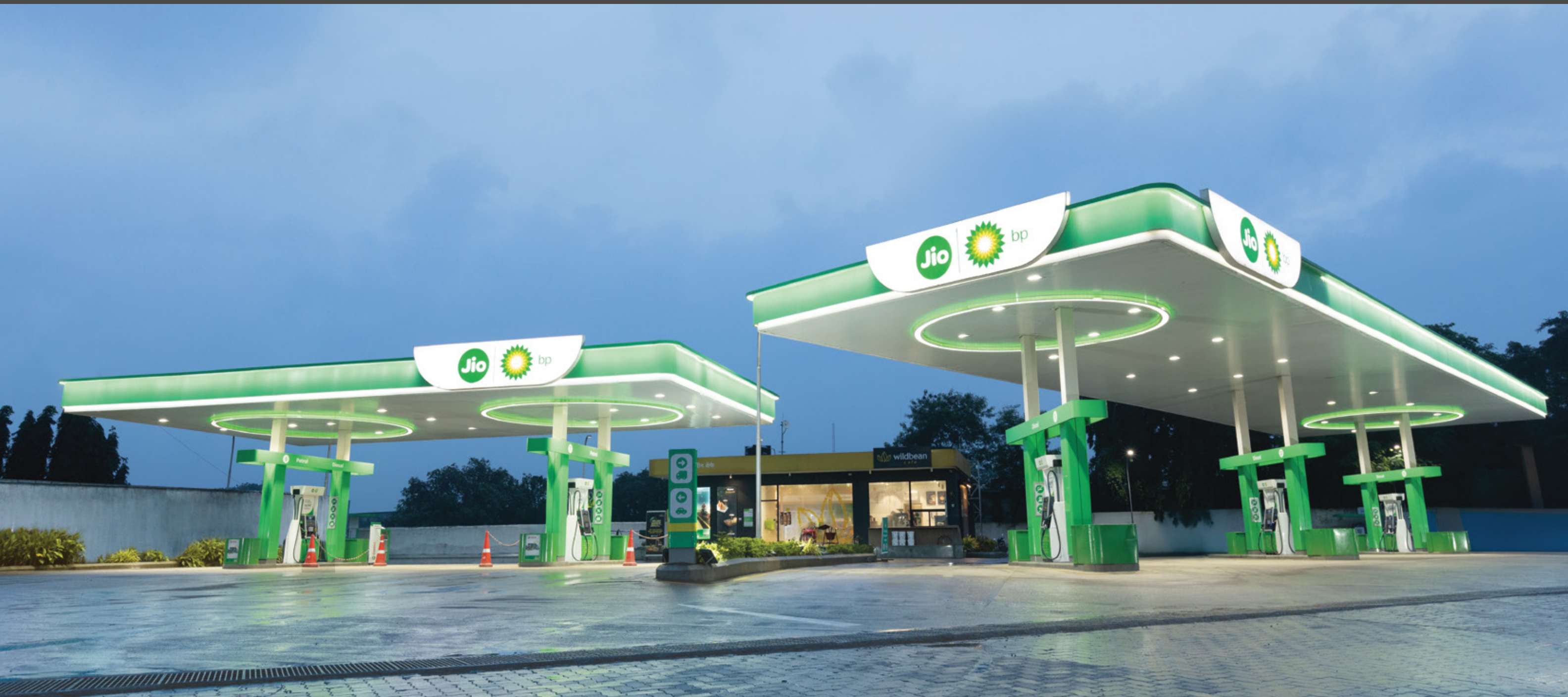
JIO-BP Petrol Station | Mumbai, India
