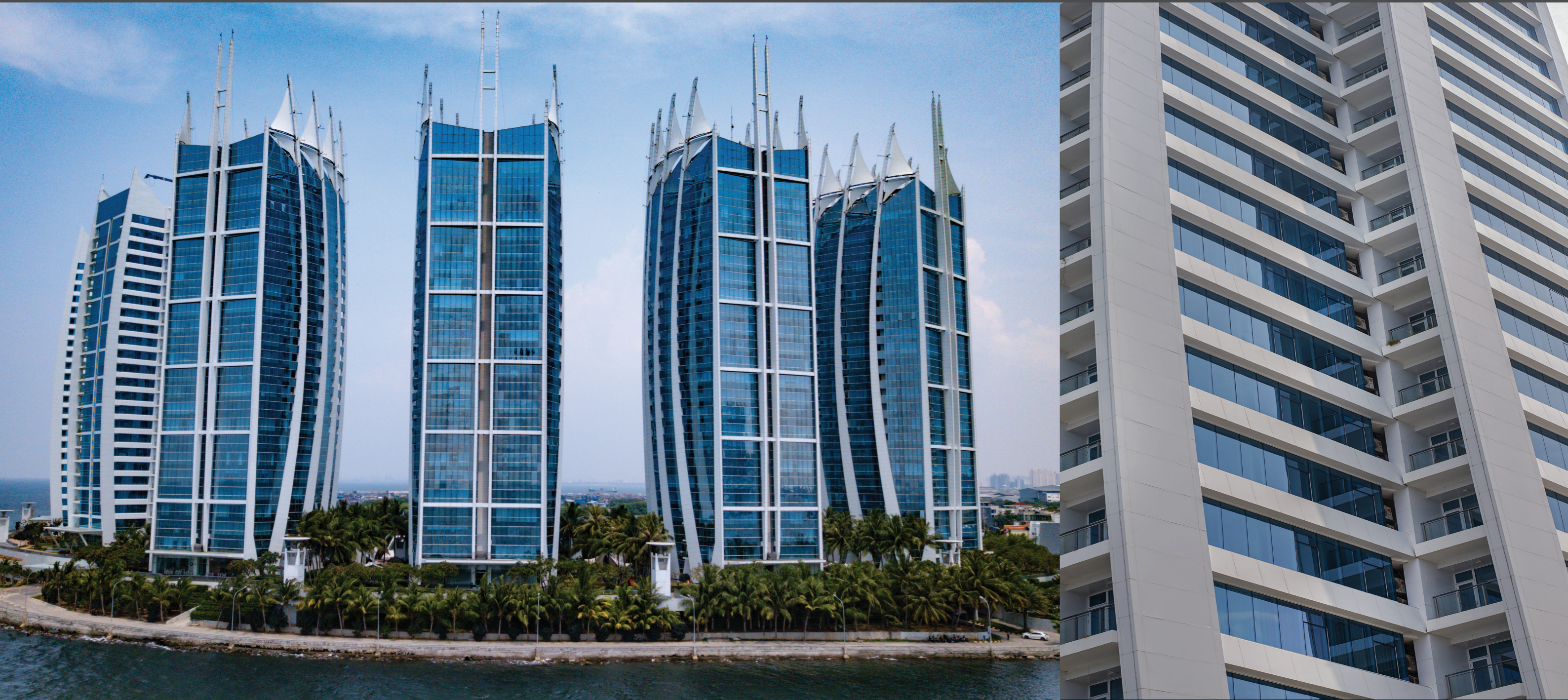
Regatta Condominium | Jakarta | Indonesia
